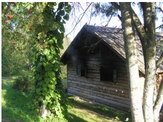
Smoke sauna, the smoke leaves the building via the windows. I am still not clear why there is no chimney.
